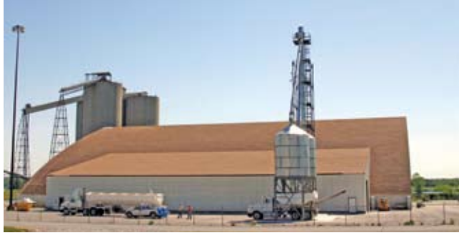
This barrel building was built in Mcleansboro, IL. It is 124 feet wide by 272 feet long and has a capacity of 27,000 tons. Internal dividing bin walls allow for multi-product storage. The enclosed blending system allows for high tonnage throughput.
